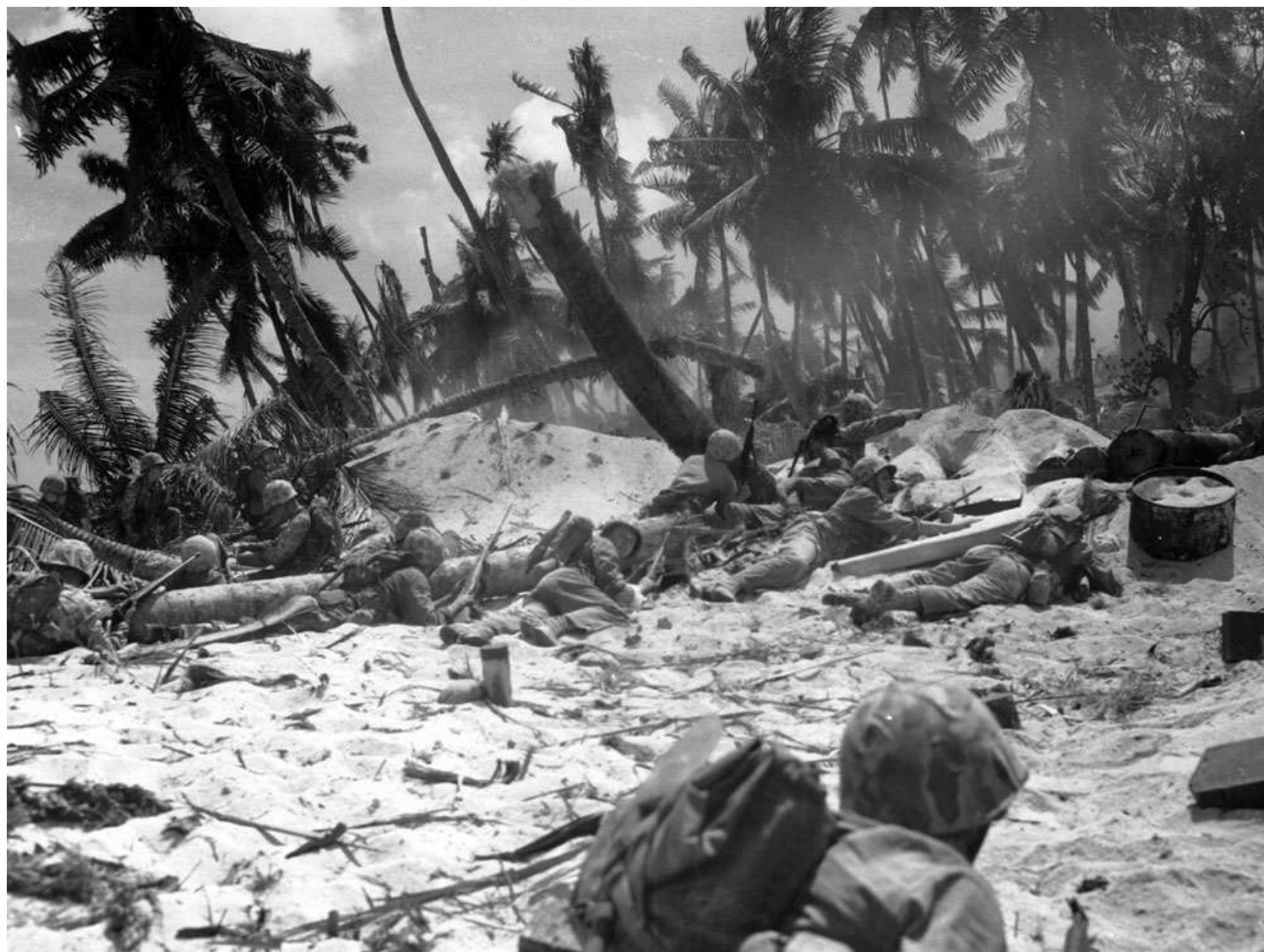
Marine reinforcements move forward across the beach at Tarawa
