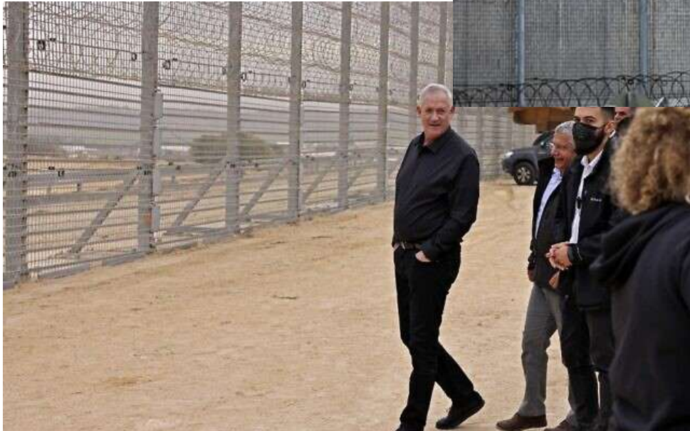
Impenetrable steel fence.
