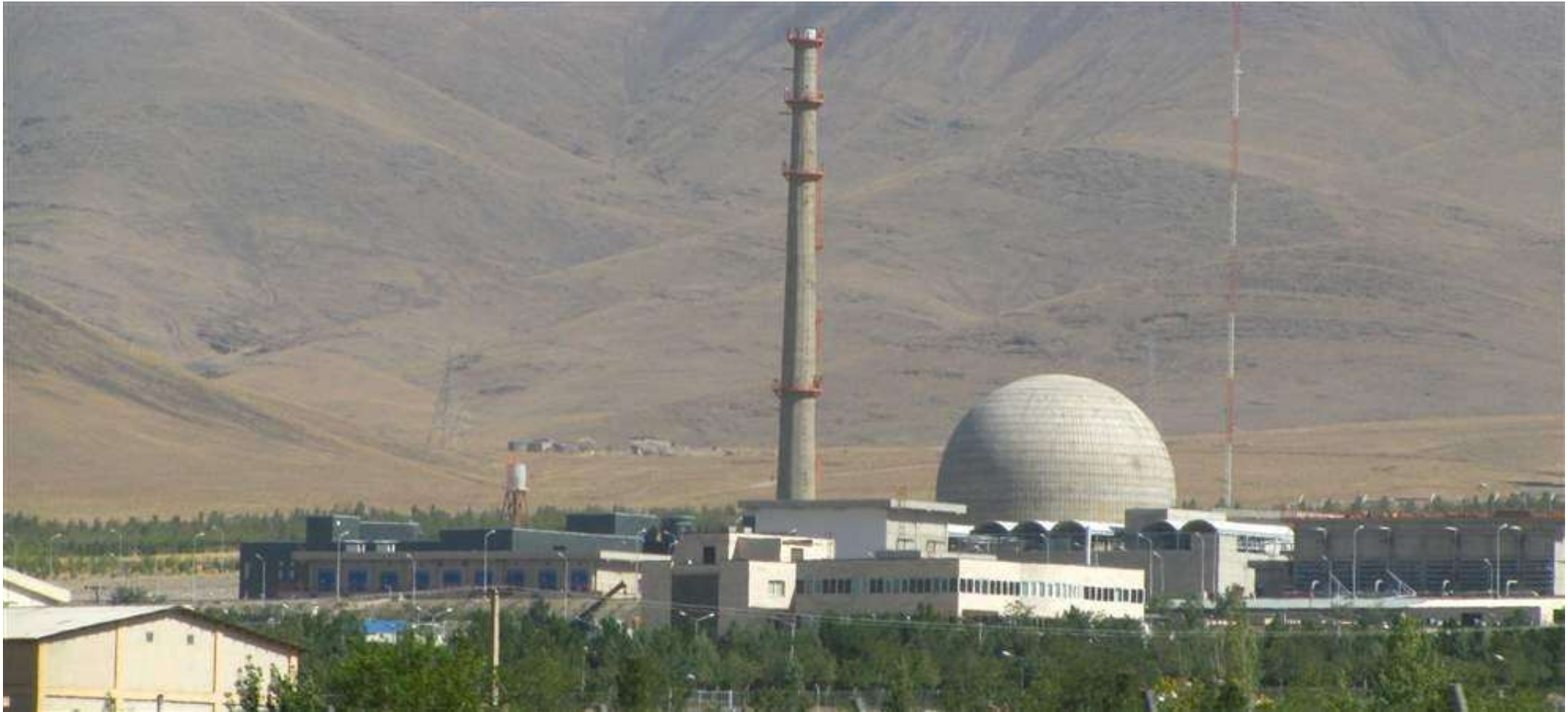
Iran's Arak heavy water nuclear plant.
