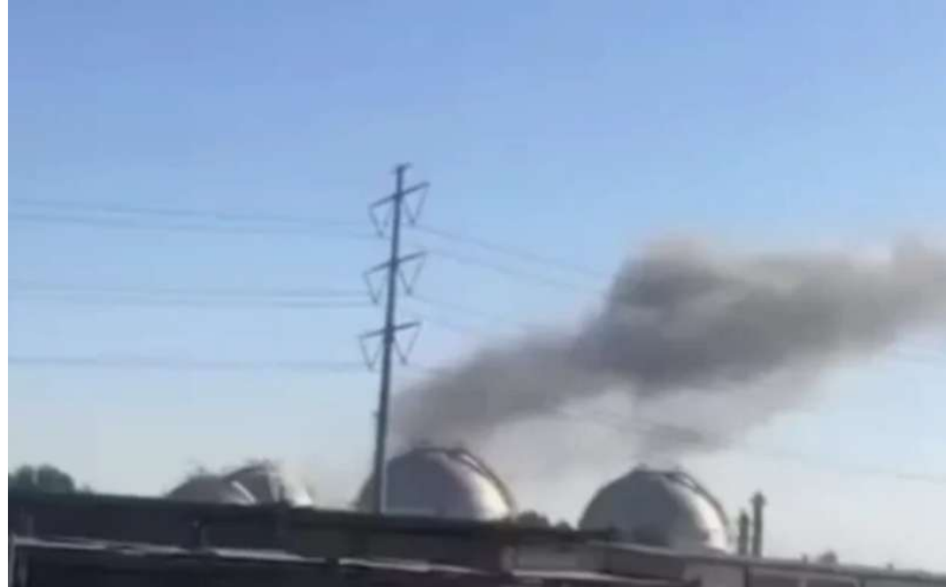
Mahshahr Petrochemical facility hit by Israeli airstrikes in southwest Iran, June 8, 2026 (Video screenshot)
